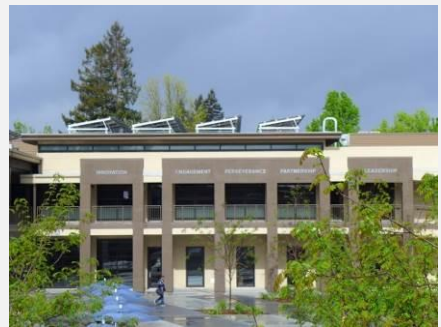
Figure 15 Solar panels on Hillview Middle School
